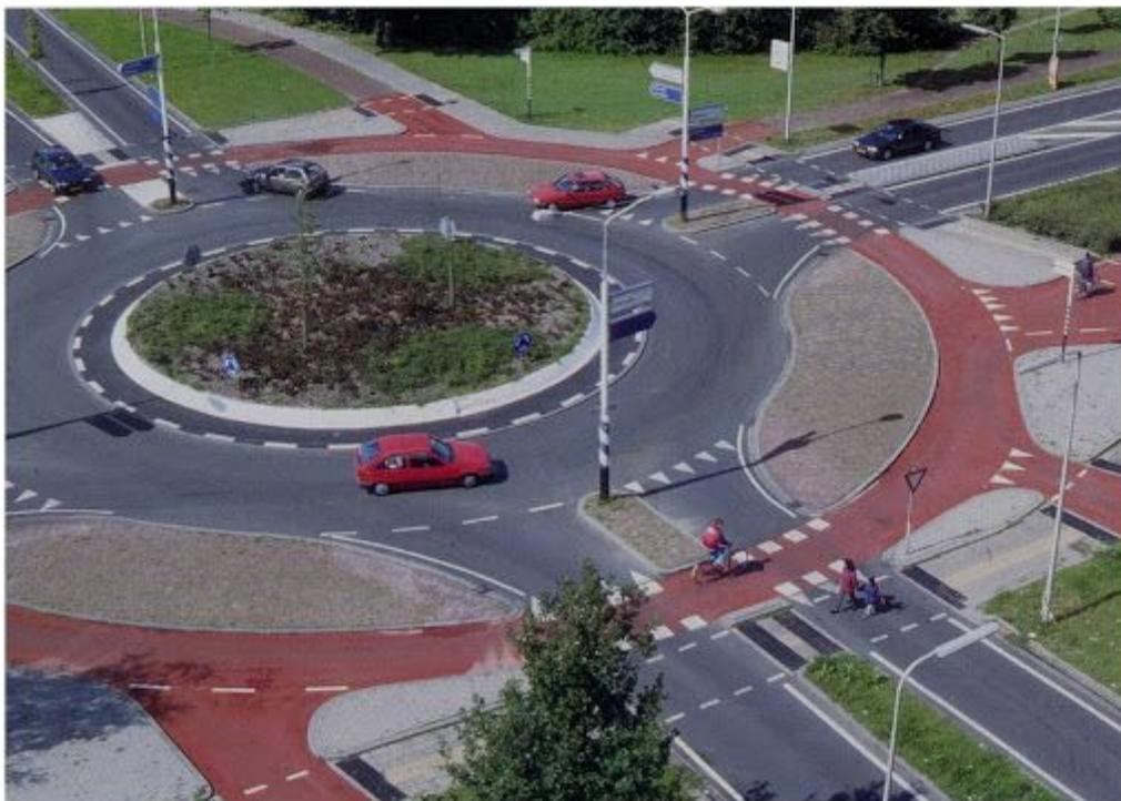
***ABOVE: FIG 2: Typical “Dutch” style roundabout. Note cyclists have a specific lane all round and priority, while traffic lanes are not very wide on approach and design ensures drivers must slow down considerably and/or stop. Cars are completely separate from cyclists except at crossings. While such designs can take up large spaces in many existing cases they can be achieved.***
